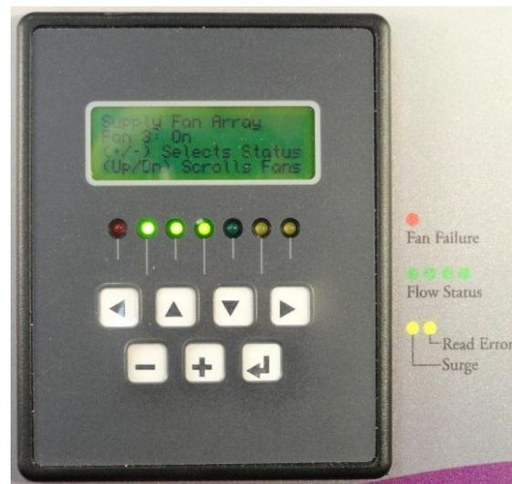
From the “**Array 1 Options**” submenu, scroll down to highlight “**7. Set Fan Status**”. Press the ↵ (enter) key and the fan status setup screen will appear. The first line on the screen will display the array name. (It should have been set in a previous step) The second line on the screen will read “**Fan 1: On**”. The number before the colon (:) is the selected fan. This can be scrolled through all of the fans in the
