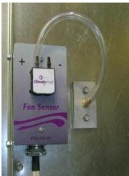
The same FSB assembly used for the fan sensor is also used for the fan array pressure rise sensor. The pressure rise sensor is mounted to the fan air seal wall on the air inlet side. The high pressure port (+) of the pressure transducer is connected to the downstream side of the fan air seal wall with flexible tubing to a bulkhead connector. The low pressure port is left open to reference the air pressure entering the fan array.
