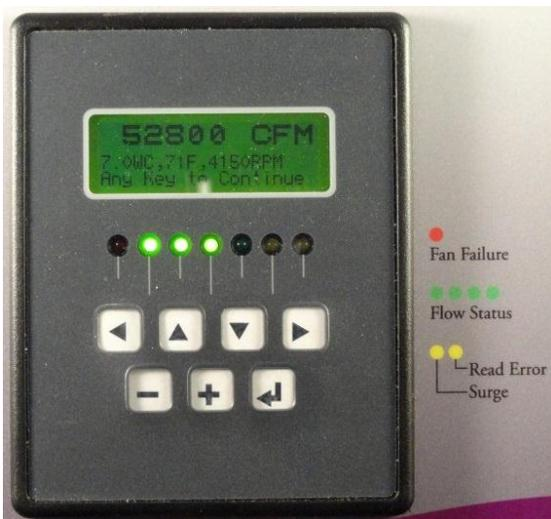
From the "Main Menu" scroll down and highlight "1. Display Airflow". This will airflow display screen. If the MatrixMonitor™ is set up for one array the following screen will appear:
