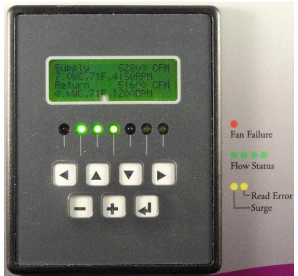
The second and third lines give the same information for fan array 2 as is shown on lines 1 and 2 for array 1.
