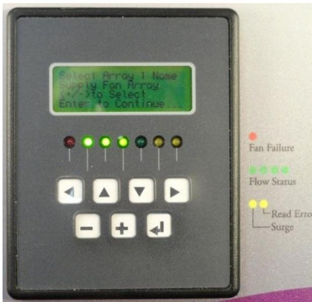
From the “Array 1 Options” submenu, scroll down to highlight “4. Array Name”. Press the ↵ key and the array name setup screen will appear. The first line on the screen will display “Select Array 1 Name”. The second line will read the array name selected from one of the labels above. The default value is “Fan Array 1”. (The default value is “Fan Array 2” for array 2). This will be displayed if the control has not been previously set up.
