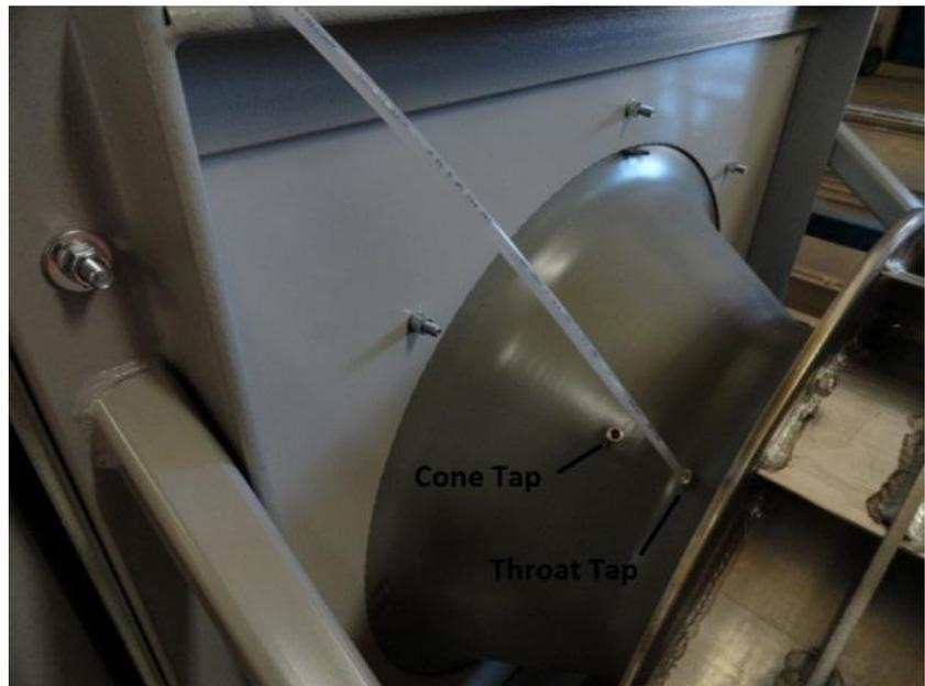
The maximum airflow in the table below is the flow at which the pressure depression at the throat or cone tap equals 13 inches WC. ClimateCraft® uses this table to select our recommended piezometric tap location. When the individual fan airflow will exceed the maximum airflow for the throat tap in the table, ClimateCraft will locate the tap in the cone. If the fan array is designed to give N-1 redundancy, the maximum design airflow will occur when one fan is off line.
