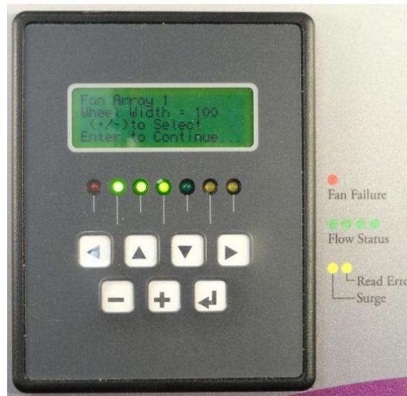
This information is available in the submittal documents for the air handling units. It will be on the fan performance data sheet. Make sure you identify the correct fan array if there is more than one in the unit.
