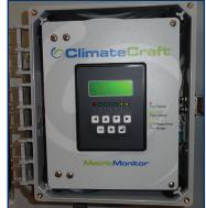
life. This package can function as a stand-alone monitoring system or it can be integrated with a building management system.
