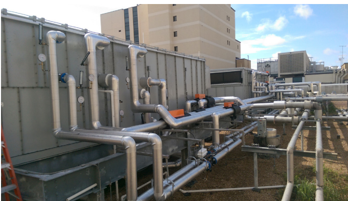
One of the three ClimateCraft custom air handlers installed on the roof of the Halifax Health Medical Center
