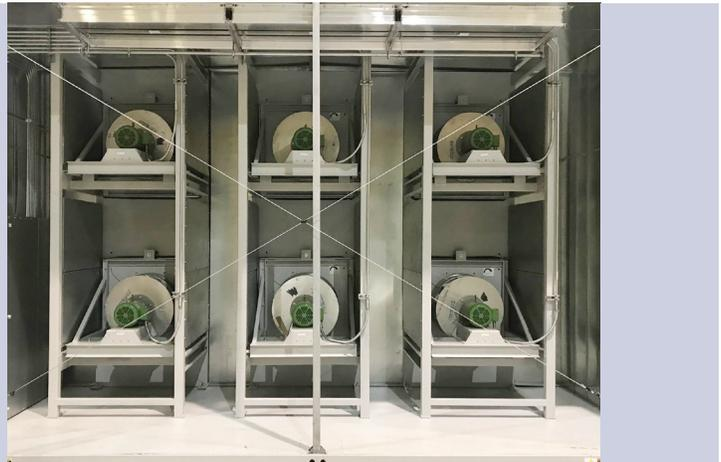
ClimateCraft's fan arrangement products allow for fans to be turned on and off for safety, repair and maintenance purposes. ClimateCraft's fan arrangement products are not designed to turn individual fans on and off for the purpose of improving fan arrangement efficiency, and ClimateCraft does not endorse turning individual fans on and off for the purpose of improving fan efficiency. Any statement to the contrary is not supported by ClimateCraft.
