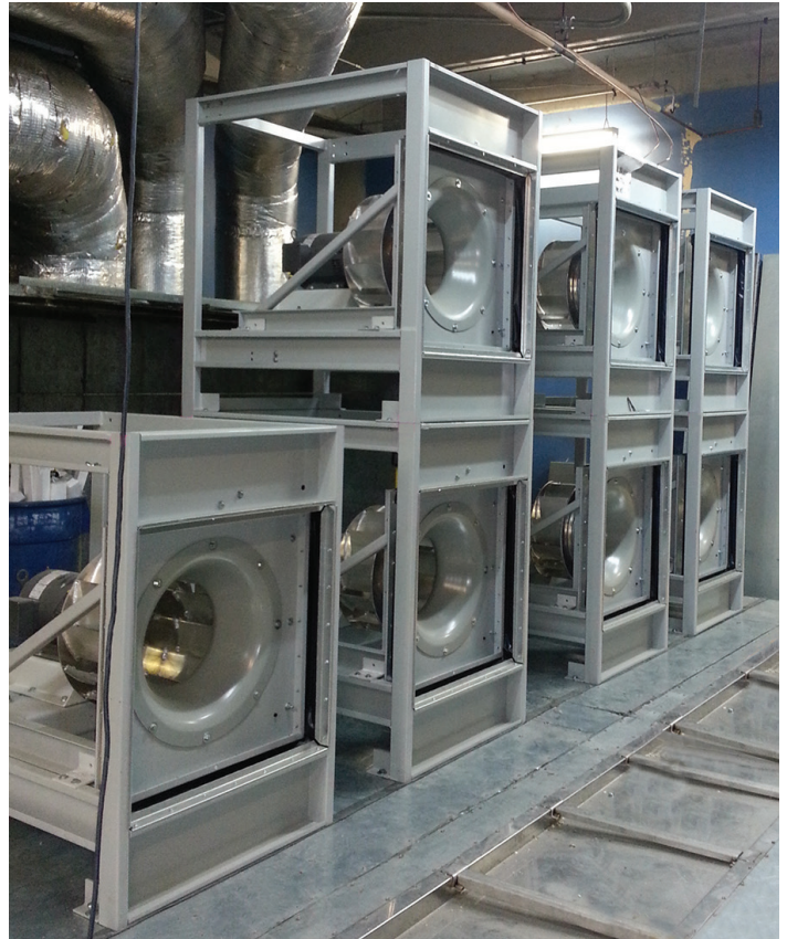
ClimateCraft FanMatrix™ fan array towers ready for installation in the site-assembled ACCESS air handling unit at Auraria Campus of the Denver Community college.
