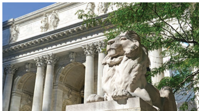
New York Public Library New York, NY 8 ACCESS site-assembled air handlers
