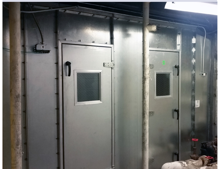
The final result—the ACCESS air handler replacement section installed and operational.
