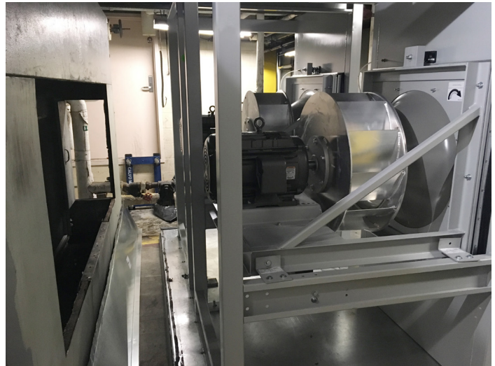
The FanMatrix™ fan array section ready for installation in the ACCESS site-assembled replacement air handler.
